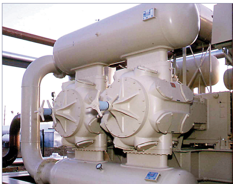
22-1/2E cylinders, 205 psig, with head-end variable volume clearance pocket unloaders.
